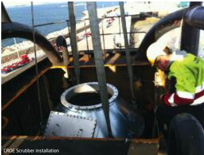
CROE Scrubber installation
